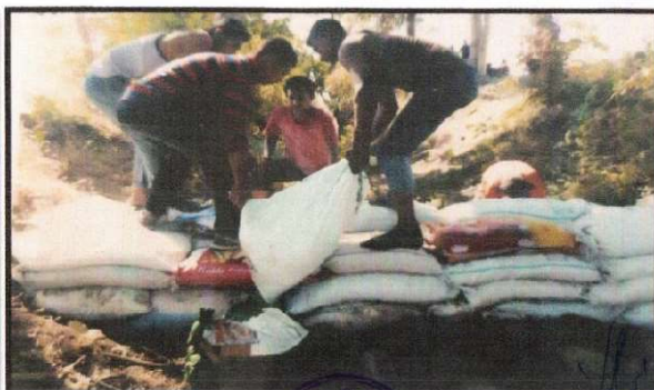
Students Building check dam under "Pani Adva Pani Jirva" Scheme
